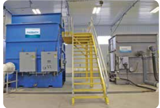
Aqua MegaDisk® (left) compared to AquaDisk® (right).
