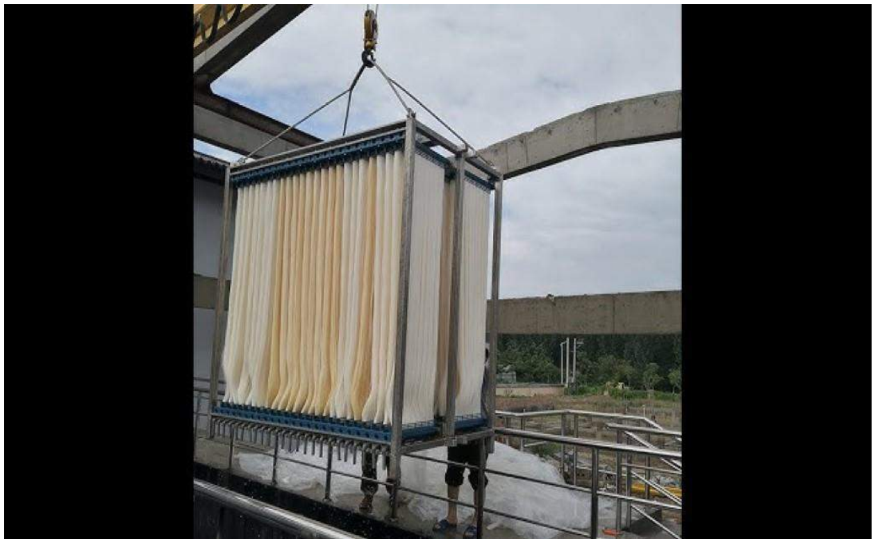
Figure 1 - Membrane units outside their basin
