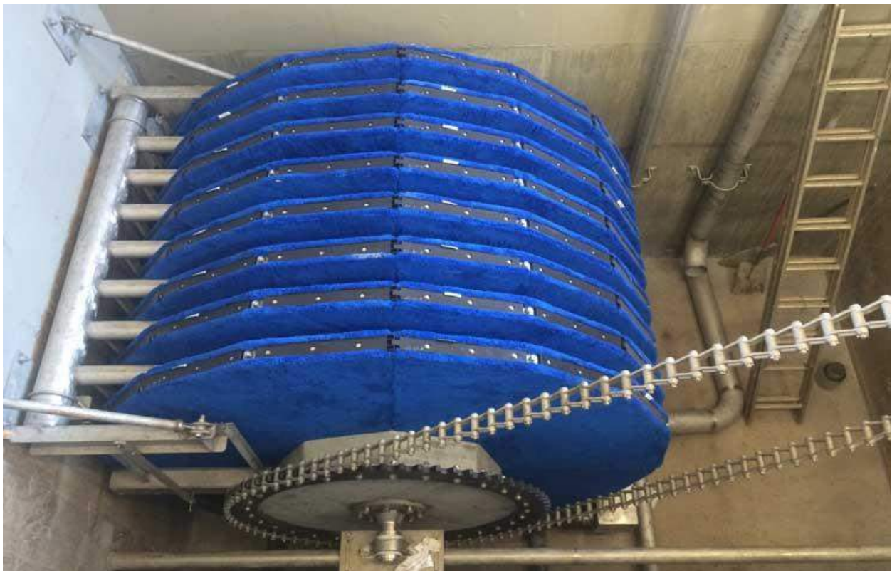
Figure 2 – Cloth disc filter unit up close
